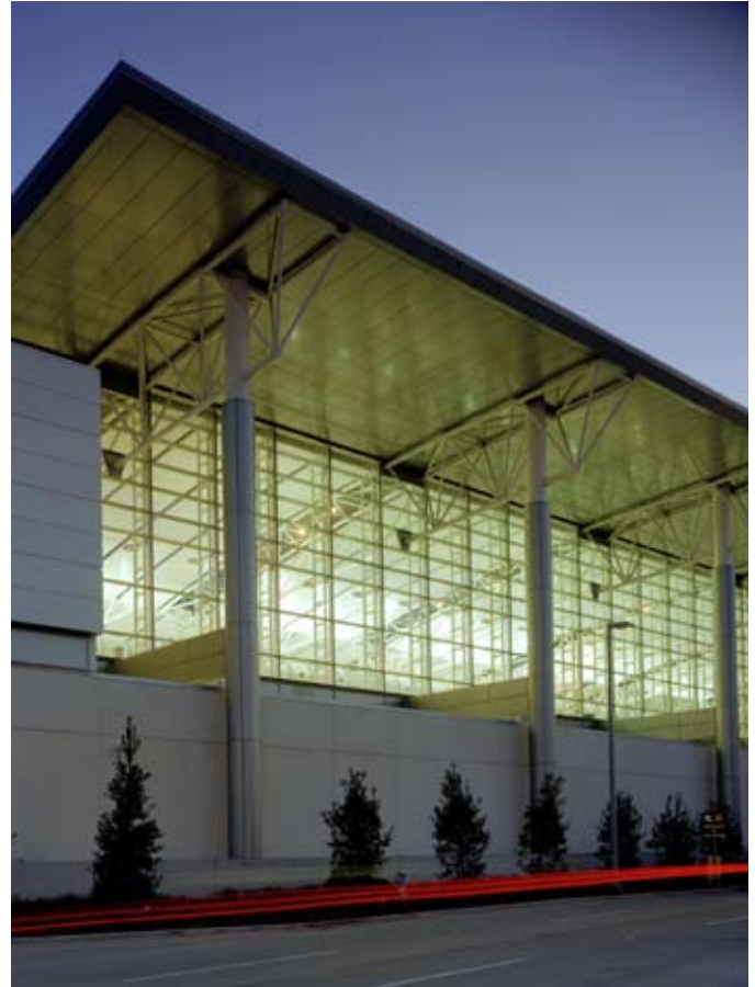
INTERNATIONAL ARRIVALS TERMINAL, GEORGE BUSH INTERCONTINENTAL AIRPORT, HOUSTON, TEXAS PHOTOGRAPH COPYRIGHT R PAYNE
