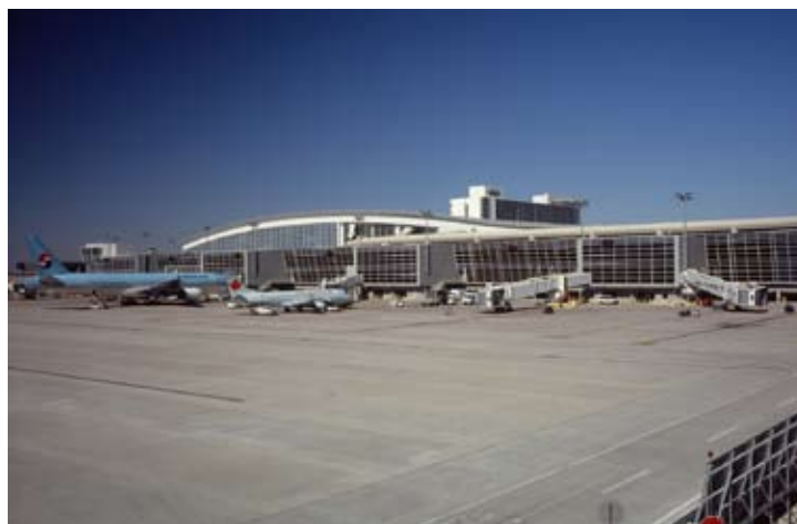
DFW INTERNATIONAL TERMINAL D, DFW, TEXAS PHOTOGRAPH COPYRIGHT WES THOMPSON
