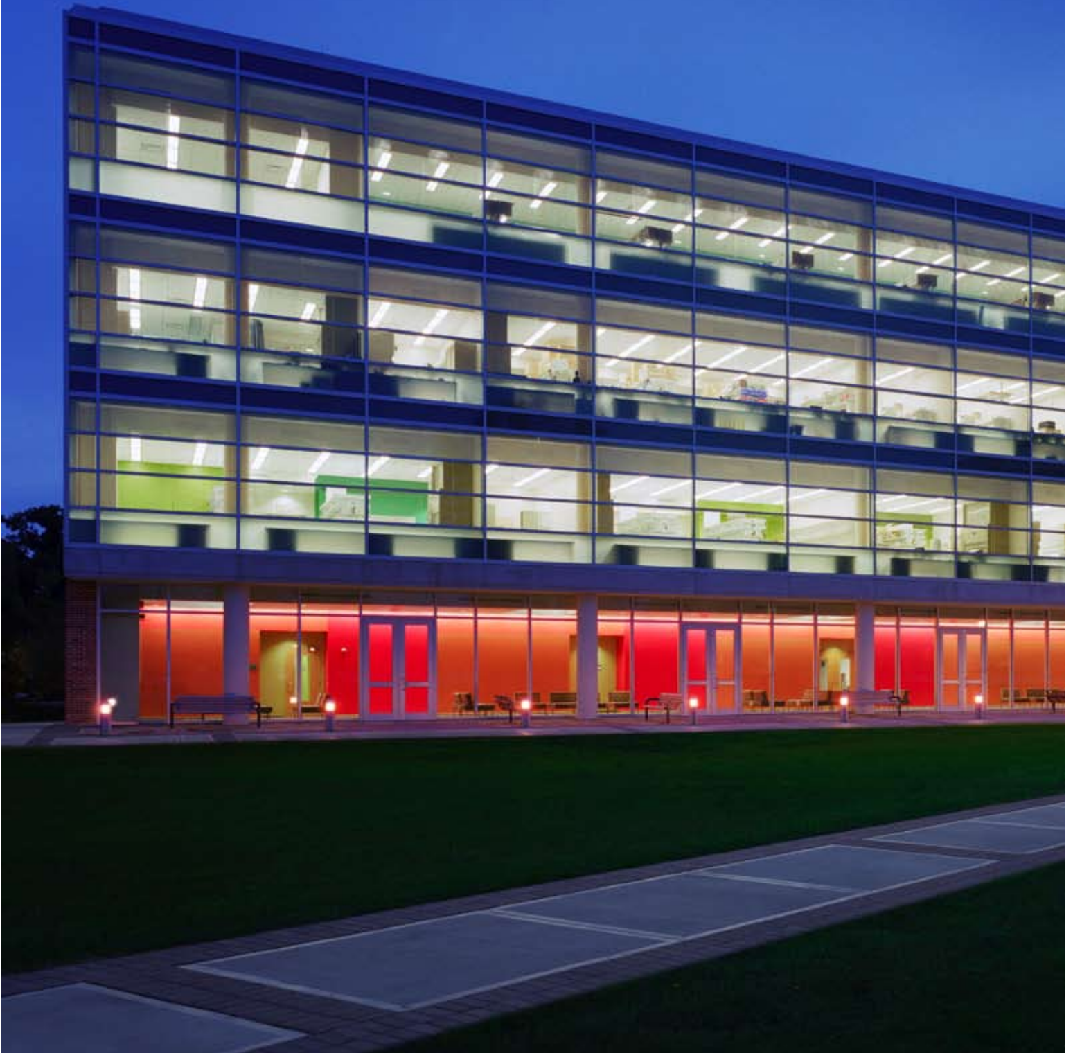
U.A. WHITAKER BIOMEDICAL ENGINEERING BUILDING, GEORGIA INSTITUTE OF TECHNOLOGY, ATLANTA, GEORGIA PHOTOGRAPH COURTESY HOK
