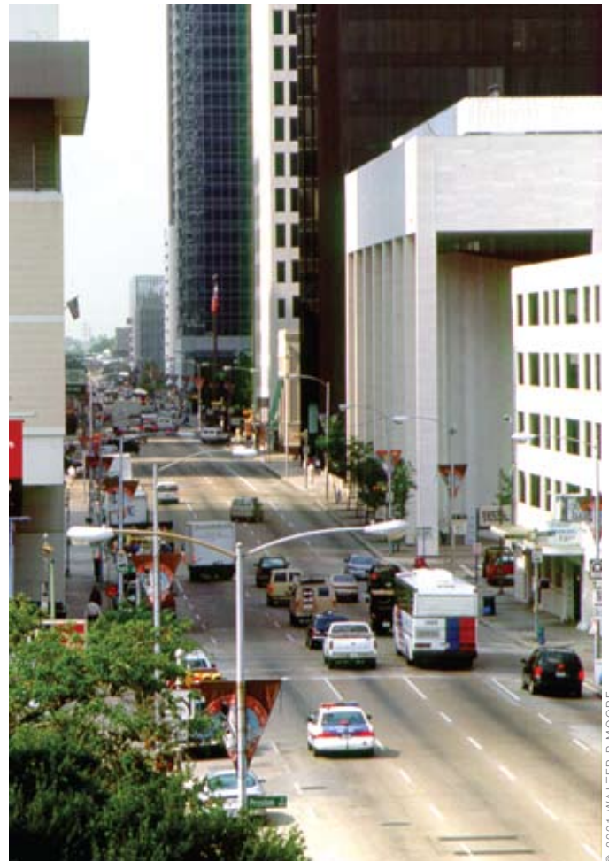
MILAM TRANSIT STREET IMPROVEMENTS HOUSTON, TEXAS
