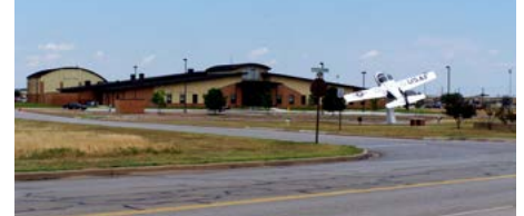
Sheppard Air Force Base Euro-NATO Joint Jet Pilot Training Program Facility, Wichita Falls, TX
