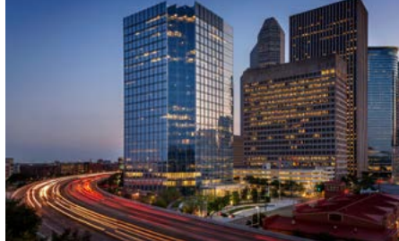
Mickey Leland Federal Building Renovations, Houston, TX
